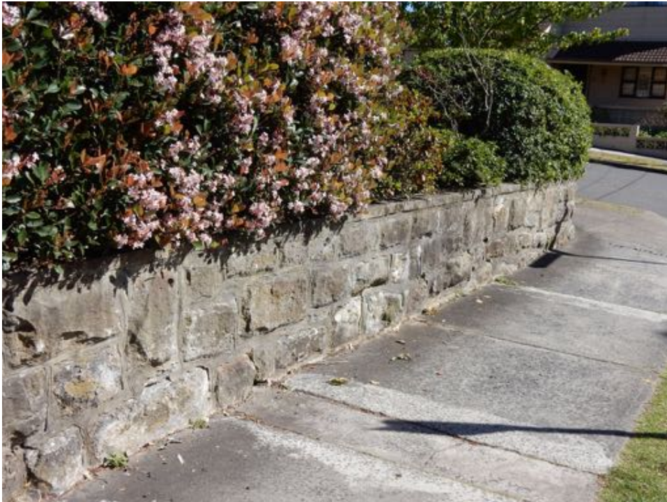
Figure 18: Sandstone retaining wall along Anderson Street boundary of 56 Anderson Street
